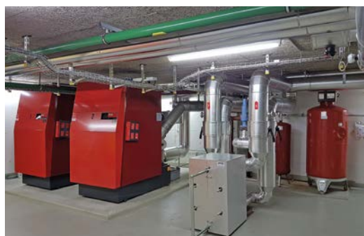
Chauffage Watt I
