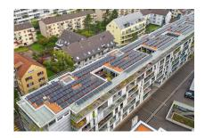
Renovation of energy systems at Dennlerstrasse 25–39 in Zurich: Renovation of electrical installations and flat roof, and construction of a 124,000 kW photovoltaic system, provision of e-mobility (Siemens) etc.
